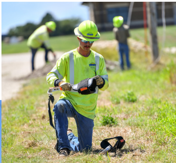
LEFT: Apprentice lineman Thomas Biery inspects a pair of lineman's hooks before climbing a pole.
